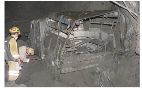
Figure 2 Property damage caused by a bulkhead failure (Fargo truck)
